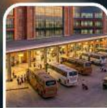
INNER STATE BUS TERMINAL
